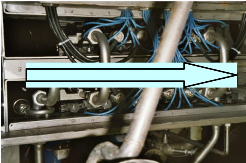
Figure 5. Top view of electrolyser (arrow indicates flow direction of dyebath)
